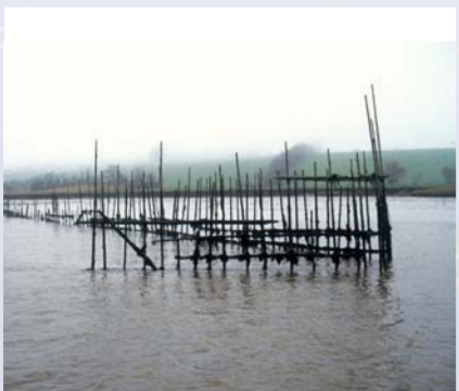
Modern tidal head weir in Waterford harbour, oriented to catch fish moving up stream or with the flooding tide. A long shore fence runs diagonally down from the shore to meet a shorter flood fence, with a raised platform situated at the eye of the trap. The Shannon estuary post-medieval and modern fish traps were broadly similar. (Aidan O'Sullivan)
