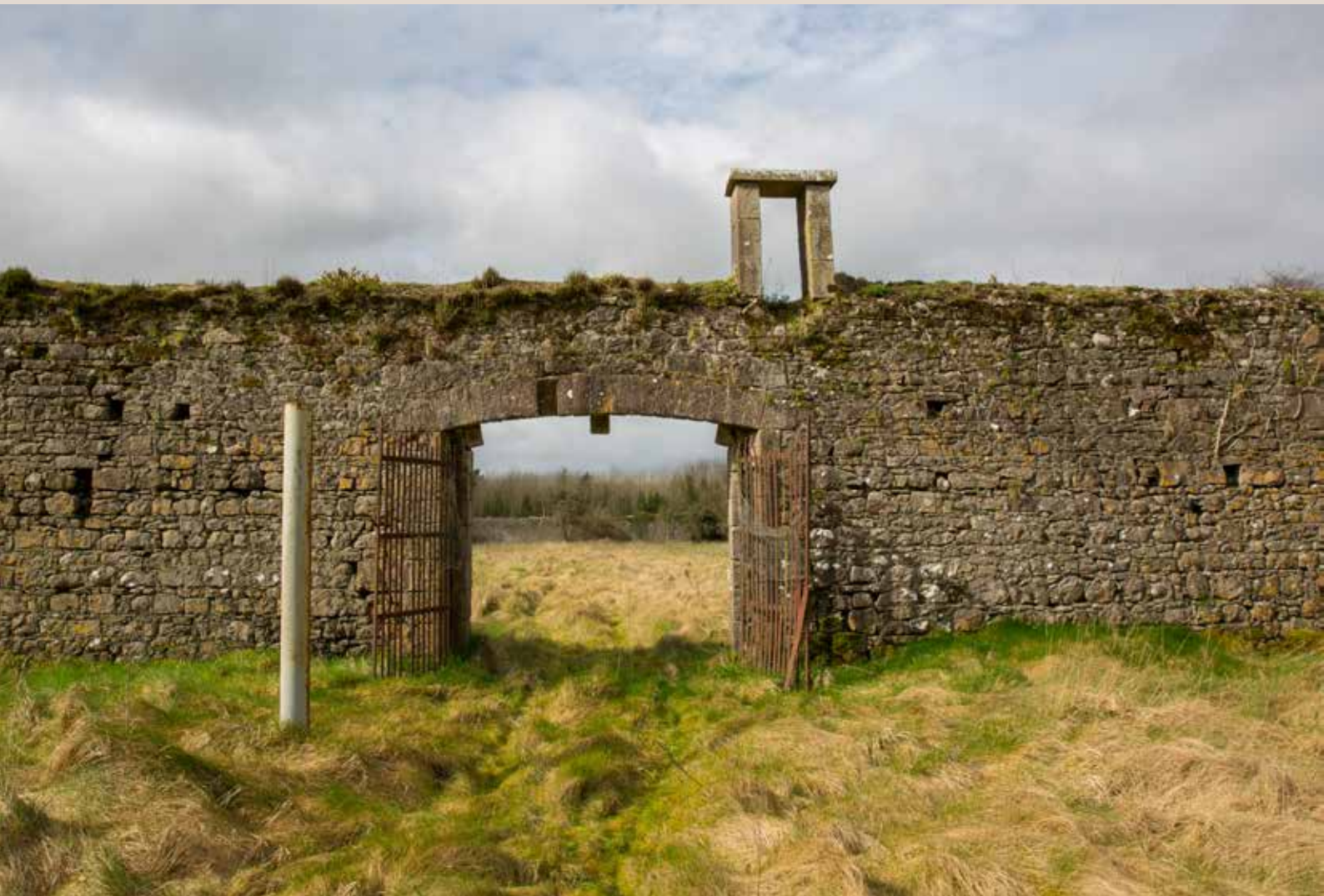
Mountbellew Walled Garden, Galway, adopted by the Mountbellew Heritage and Tourism Network 2017
